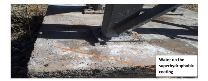
The polyurethane superhydrophobic coating has two components that should be mixed together before applying on the surface. It can be applied by brush, rolls and spray gun. The coating will be cured in room temperature after 12 hours. The coating was confirmed by York University in Canada.
